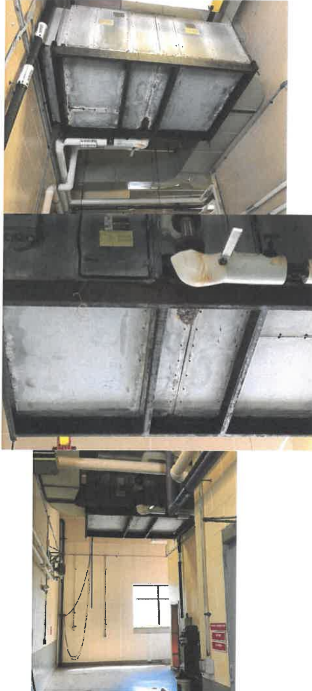
Air Handling Unit to Be Replaced
