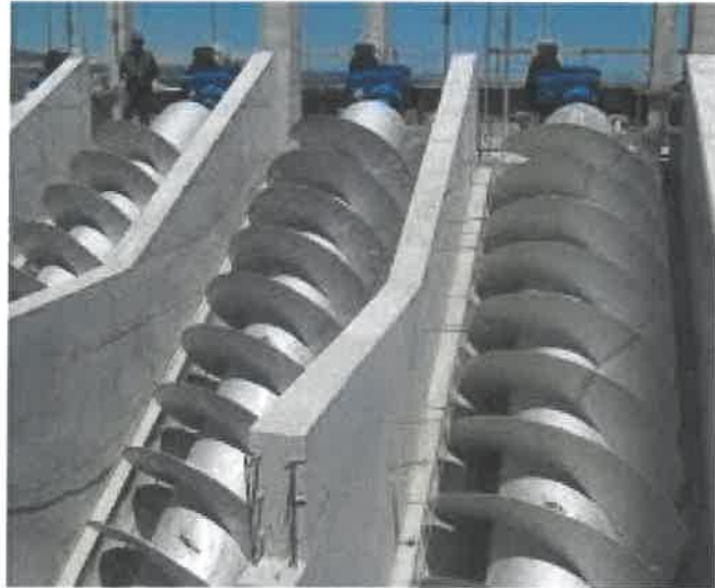
Sample Picture of Screw Pumps to be Replaced
