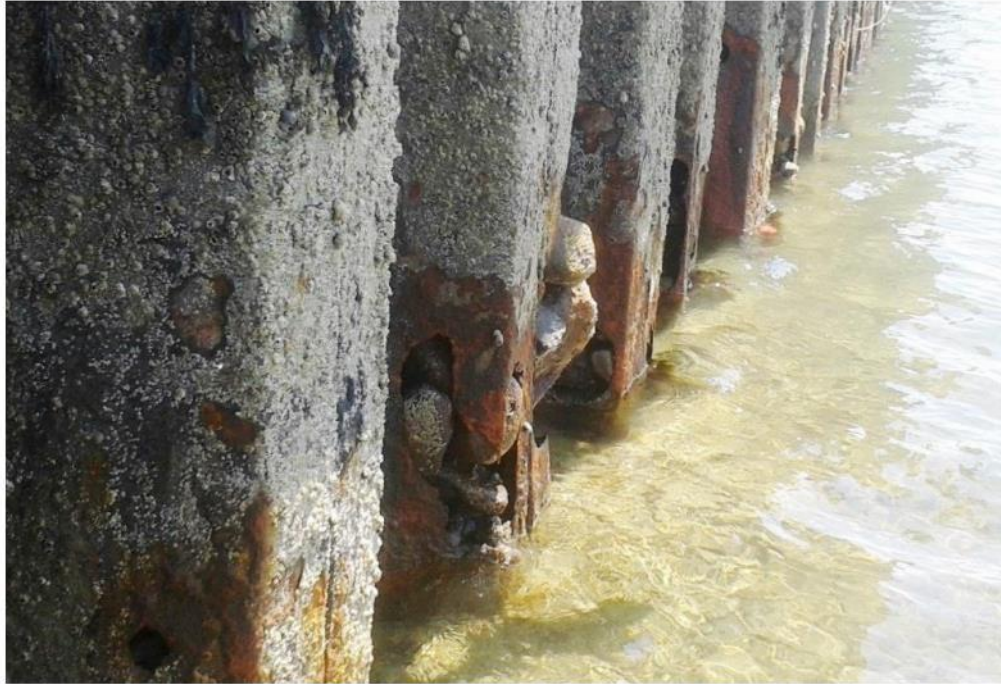
Photo 7 Southern park area bulkhead view at low tide in the vicinity of the fence line. Note numerous corrosion holes and apparent loss of backfill
