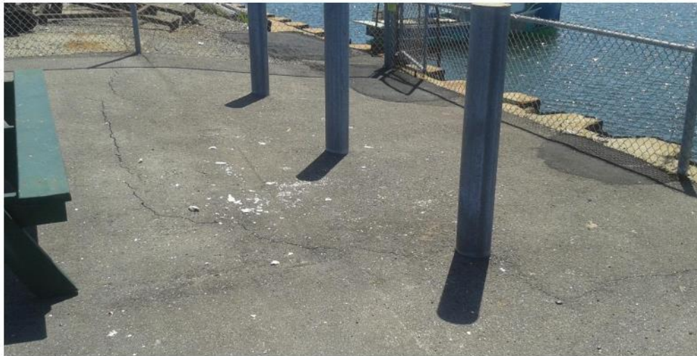
Photo 8 Southern park area bulkhead in the vicinity of the fence line. Note pavement crack parallel to bulkhead at 12 to 13 feet back from sheet piling indicating a larger area of backfill subsidence is starting. A recent looking pavement patch has also been added on the fisherman's coop side of the fence.
