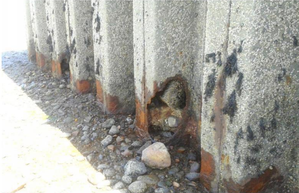
Photo 3 Northern bulkhead area showing low tide level corrosion holes in the sheet piling and likely source of backfill wash-out
