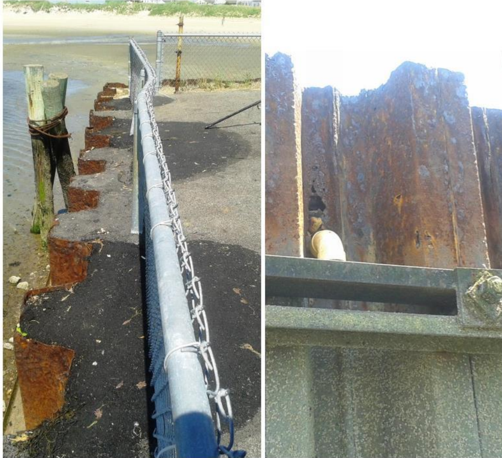
Photo 2 Northern bulkhead area showing recent pavement patches and corresponding corrosion holes in the sheet piling upper "splash zone" area. Note some subsidence of one railing post into the middle sinkhole
