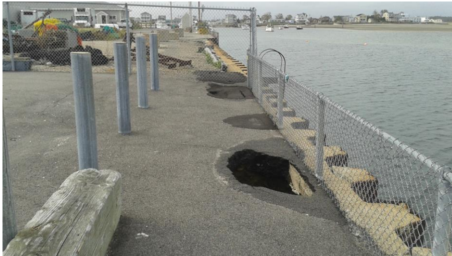
Sinkholes observed on landing / loading area adjacent to bulkhead.
