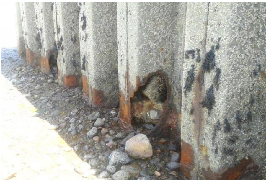
Northern bulkhead at low-tide showing corrosion in the sheet piling, one likely source of backfill wash-out.
