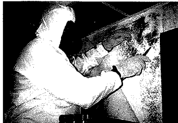
Take steps to protect yourself. Use an N-95 or equivalent dust mask, rubber gloves, eye goggles, and disposable clothing.
