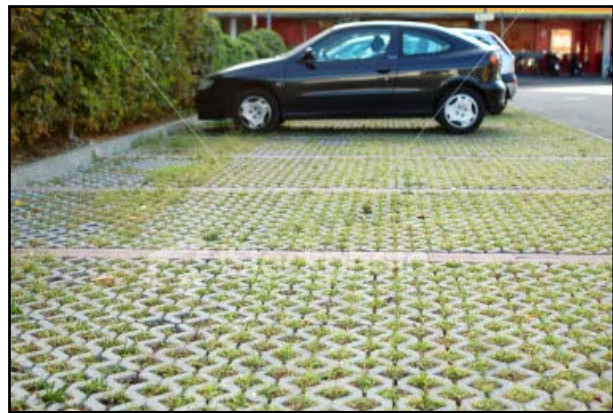
Paver grids in light-duty parking areas are installed with a soil medium that supports plant growth and infiltrates runoff.
