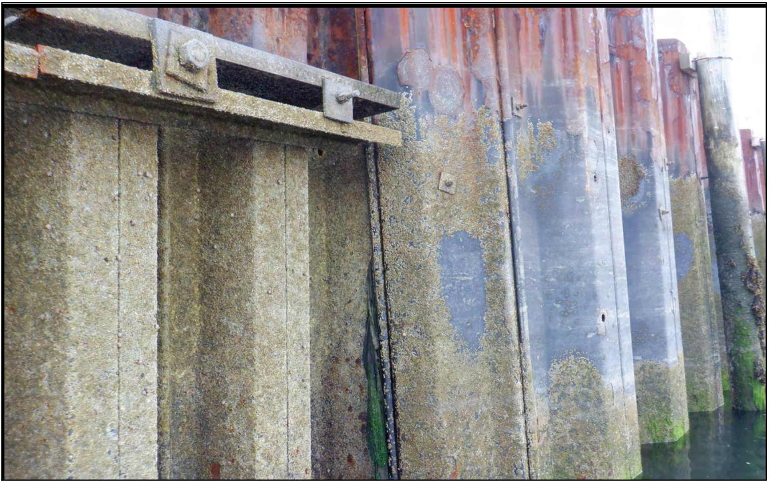
6 – PREVIOUS BULKHEAD REPAIR TRANSITION, LOOKING SOUTHEAST
