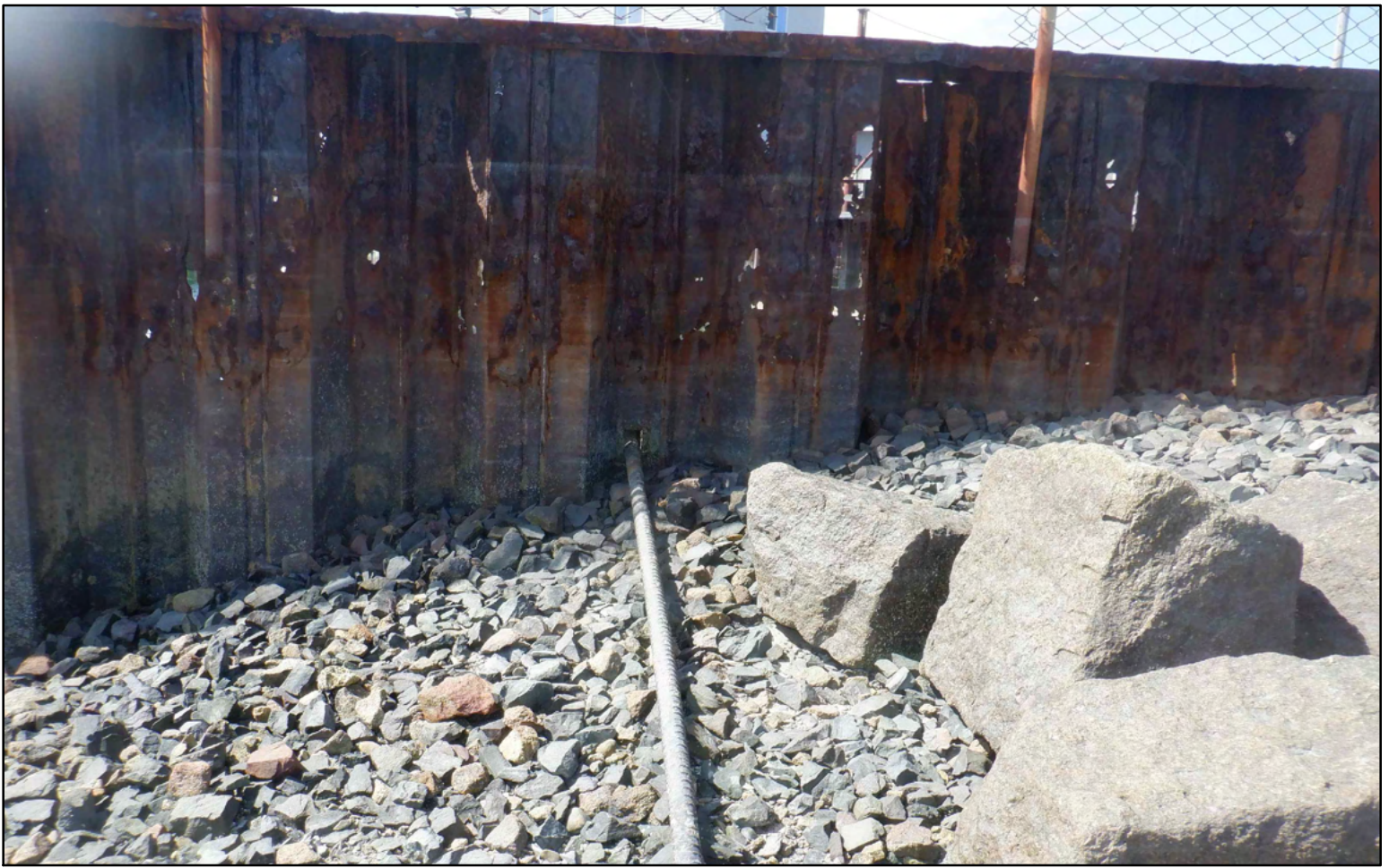
9 – EXPOSED TIEBACK SYSTEM AT SOUTH BULKHEAD, LOOKING NORTH
