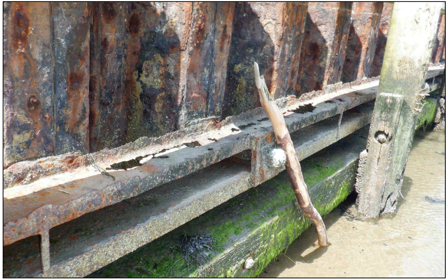
5 – TYPICAL WALE CONDITION ALONG NORTH BULKHEAD, LOOKING WEST
