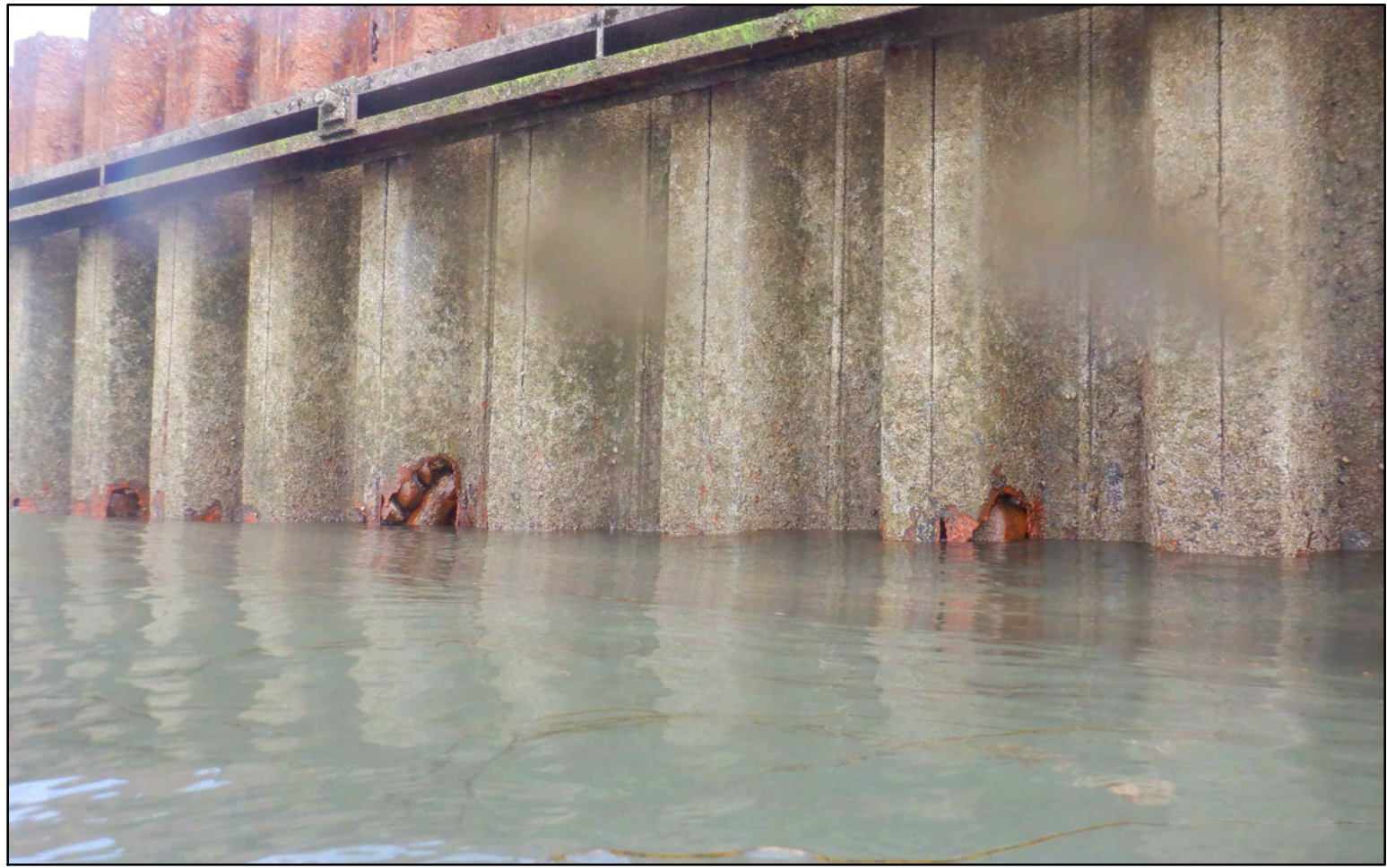
4 – CORROSION HOLES NEAR MLW, LOOKING NORTHEAST
