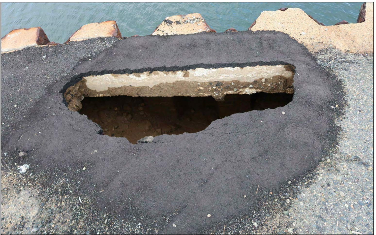
3 – TYPICAL SINKHOLE ALONG NW BULKHEAD, LOOKING DOWN
